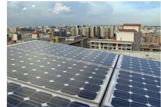
Solar panels on rooftops of HDB apts.
