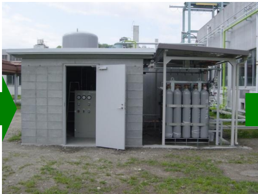
Compressor & Gas holder
